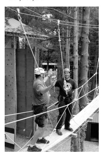
The Ewok Bridge consists of a pair of foot cables that support a horizontally positioned wooden foot bridge. The bridge includes two Multi-line rope hand rails.
